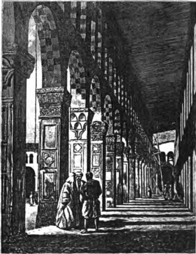
ORNAMENTED PIERS AND ARCHES IN THE COURT OF THE GREAT MOSK
