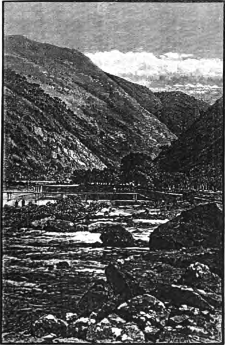
THE WEIR ACROSS NAHR EL KELB.
