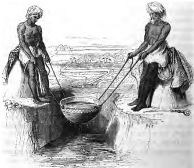
[Irrigation by the Ckutweh.]
